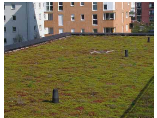
Grønt tak (Scharnhauser Park, Stuttgart).
